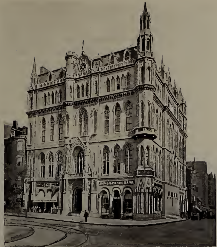
MASONIC TEMPLE, Tremont and Boylston Streets. Electrical construction work by the Lord Electric Co., 181 Tremont Street.
